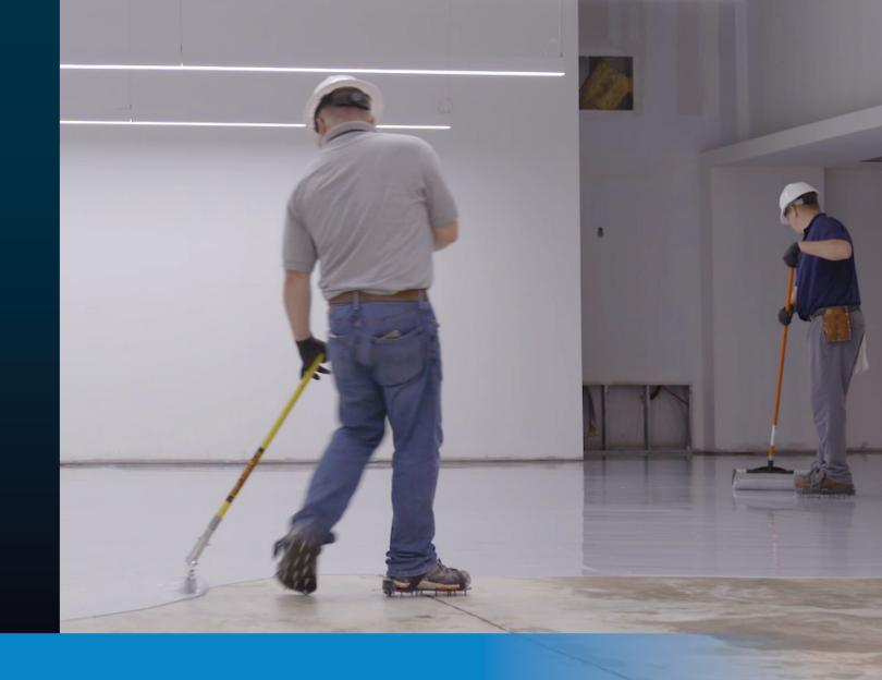
Poured moisture barrier on prepared surface
